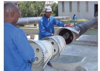
Drag trowel process
