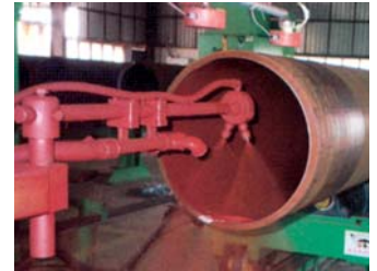
Application of liquid epoxy
