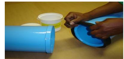
4. The gasket is pushed back over the joint so that the two lips of the gasket each rest on the shoulder end and that no part of the gasket extends over the pipe shoulder. Remove one bolt and slacken the other to allow the coupling to swing over the joint. Fit the coupling halves over the gasket to position the housing key sections over the pipe shoulders.
