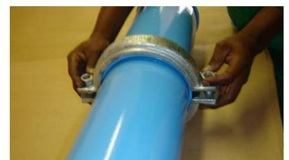
6. Tighten until the coupling halves are firmly together – metal to metal. Do not exceed the recommended maximum torque value. A ratchet wrench with an adequate output torque is recommended for this application.
