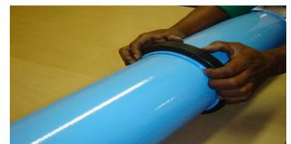
5. Insert the bolt and ensure that the oval neck fits correctly into the bolt hole and finger tighten the bolts. Tighten the nuts alternately and uniformly; maintaining an even gap between the coupling halves all the time ensuring that the gasket is not pinched.
