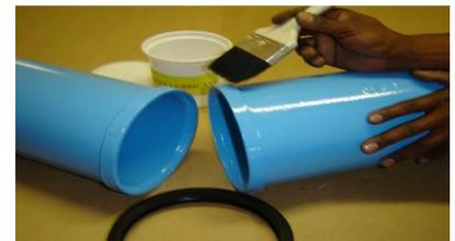
3. Ensure that the gasket is suitable for the intended use. Lubricate the gasket with a suitable non-petroleum based lubricant. The gasket is slid completely onto one of the pipe ends. The other pipe end is pushed together against the fixed one and is aligned both horizontally and vertically. Do not use the coupling during installation to align the pipe.
